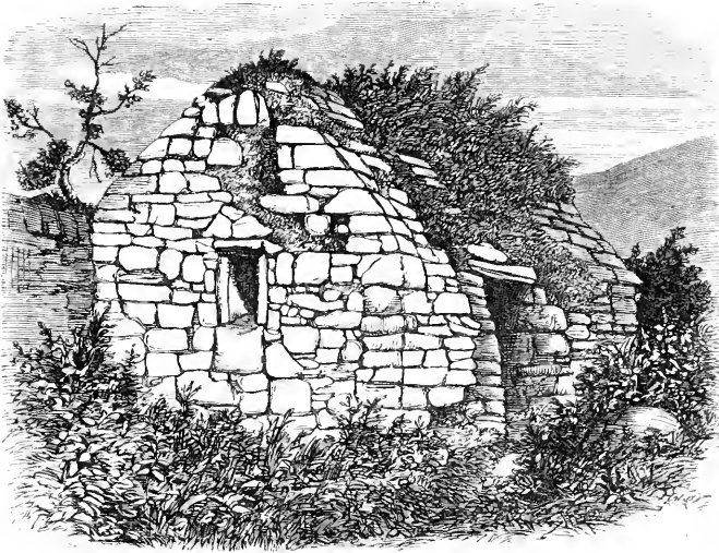
Fig. 7. Eastern gable and north side of the building.
